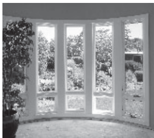
Paul received assistance from both Truitt & White and Marvin Windows, who worked with a CAD specialist that created a life-size drawing of the windows to ensure precision installation in the curved wall.
